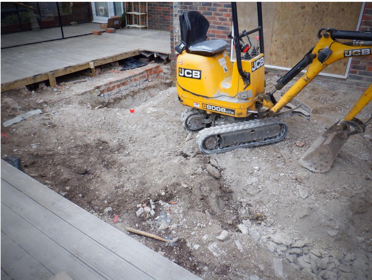
Plate1. Removal of internal concrete floor
